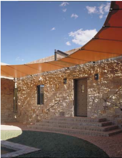
FIGURE 3 Burnside Courtyard Close Up
