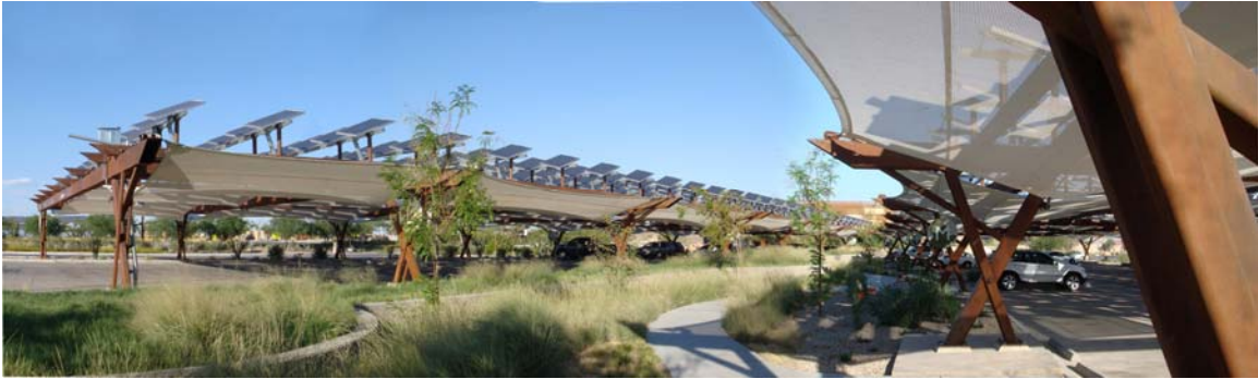
FIGURE 7 Springs Preserve Photovoltaic Parking Covers
