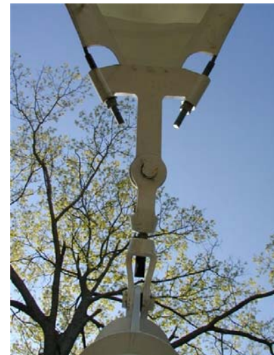
FIGURE 6 Springboro Mast Top Connection
