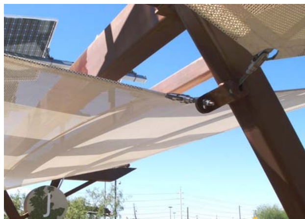
FIGURE 10 Intermediate membrane & valley cable attachments
