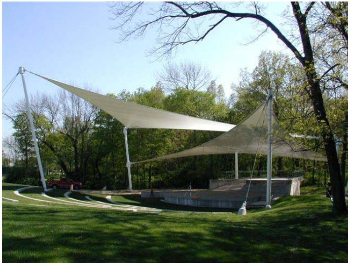
FIGURE 5 Springboro Amphitheater Canopies
